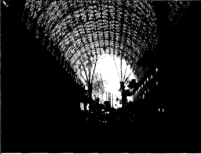
The Vault at Freemont Street
