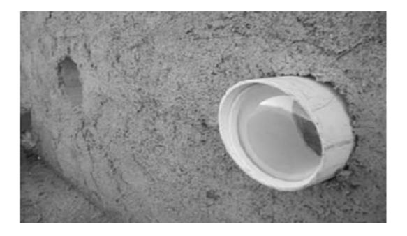
Image 6. Window made of a sewer pipe and a dinner plate set in papercrete wall
