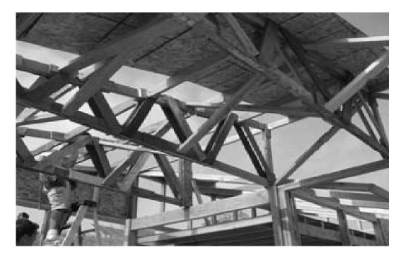
Image 5. Wood pallet roof truss system
