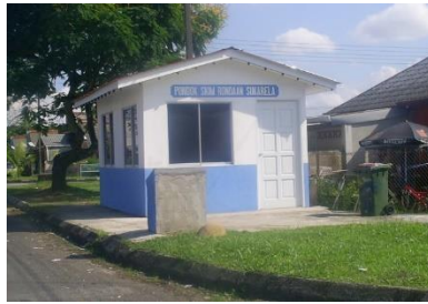
Figure 1: Community guard house
